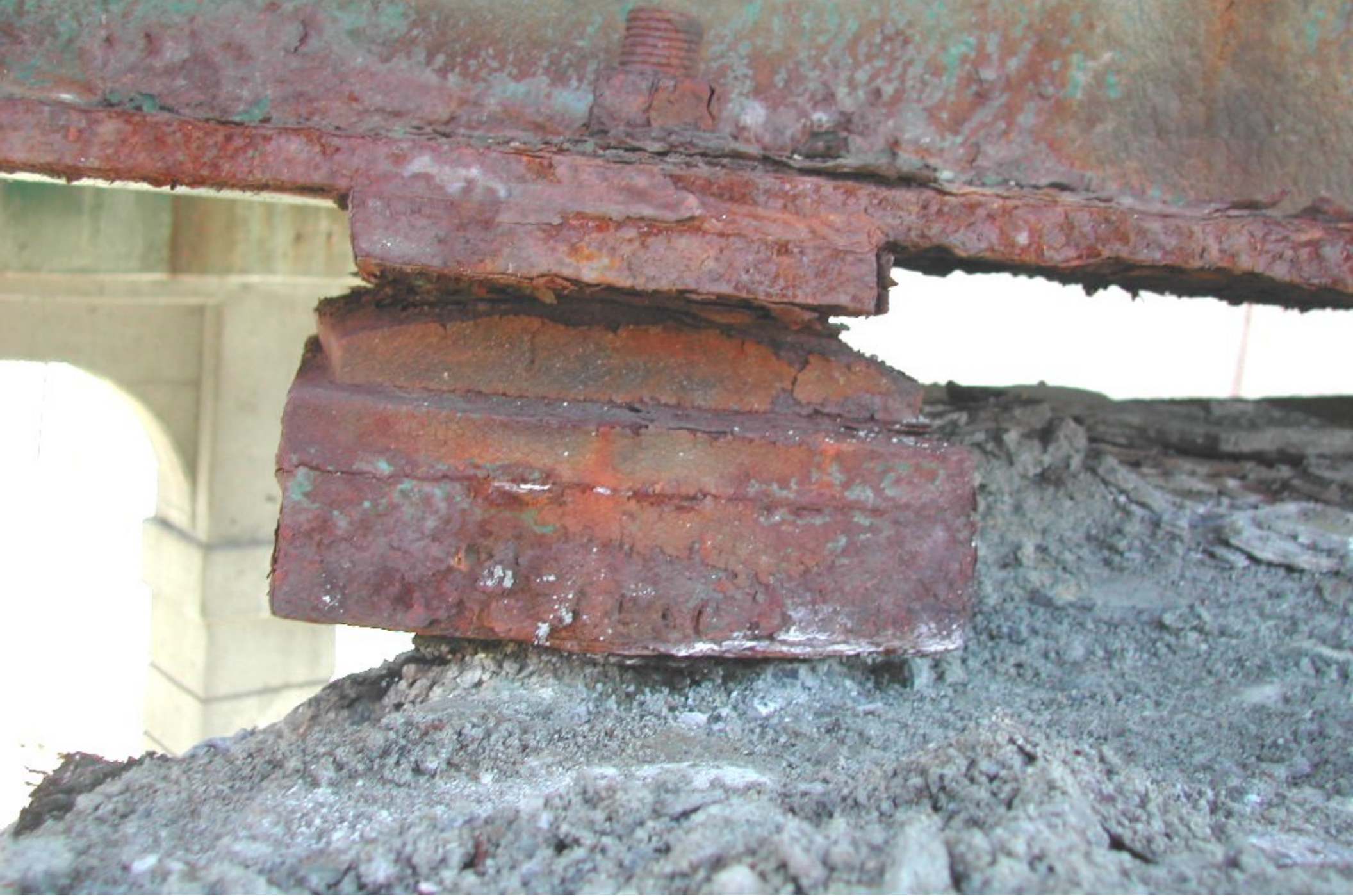
Bearing #1 at northwest corner of pier #1
