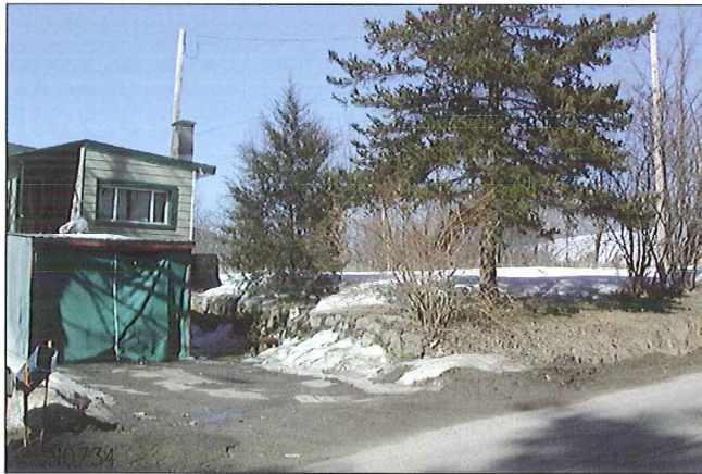
LOOKING FROM SOUTH TO WEST NOTE: DRIVEWAY IS CUT IN TO NEXT ROAD. WOULD ACCOMODATE RAISED PROFILE.
