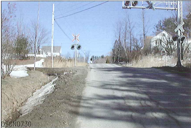
LOOKING FROM SOUTH TO NORTH SUBSTANTIAL UPGRADE
