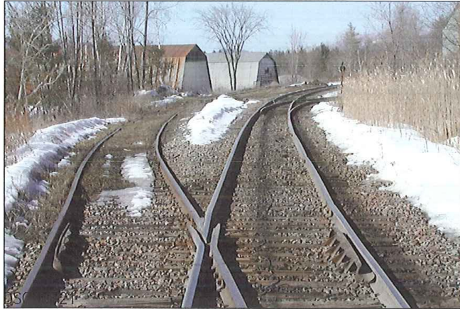
LOOKING WEST FROM WEST SIDE OF CROSSING MAINLINE ON RIGHT
