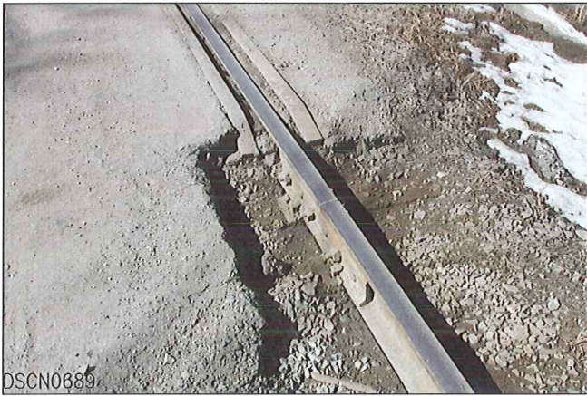
NORTHEAST CORNER OF CROSSING WELD REPAIR
