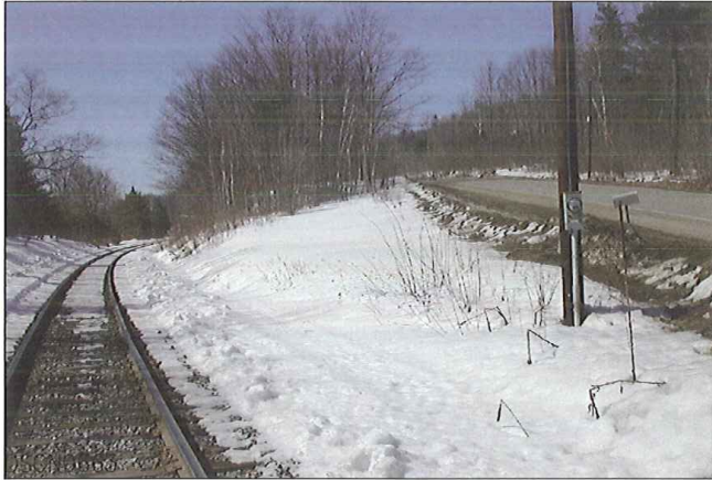
LOOKING FROM WEST TO NORTH
