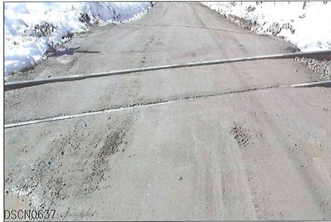
LOOKING FROM NORTH TO SOUTH SHARP GRADE BREAK
