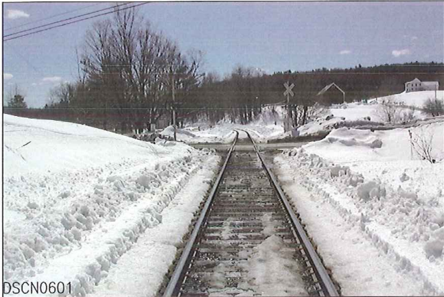
LOOKING FROM WEST TO EAST
