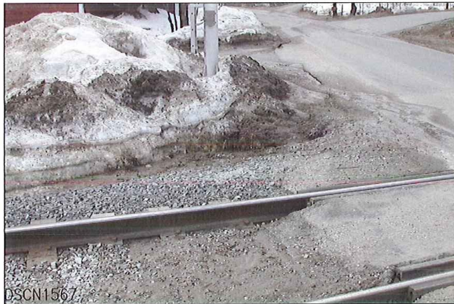
LOOKING FROM NORTH TO SOUTH, EAST SIDE OF CROSSING
