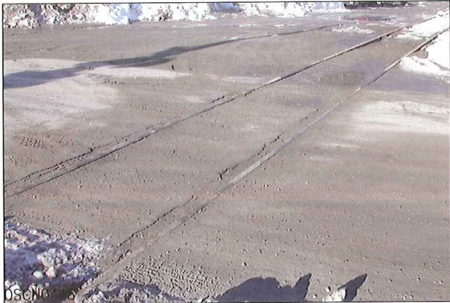
LOOKING FROM EAST TO WEST SIDE TRACK
