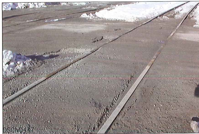
LOOKING FROM EAST TO WEST MAINLINE IN FOREGROUND
