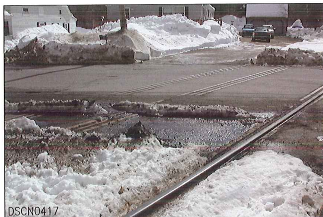
LOOKING FROM EAST TO WEST MAIN LINE & SIDETRACK
