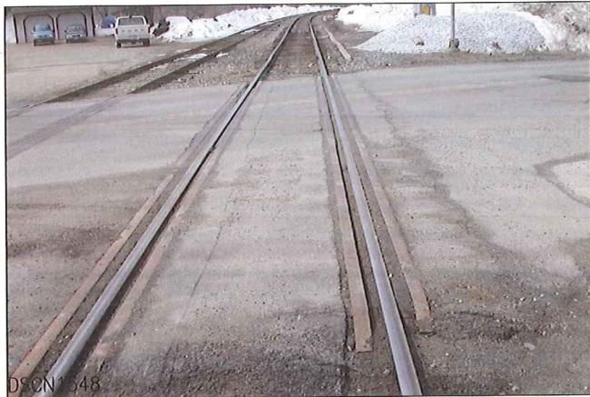
LOOKING FROM EAST TO WEST, MAINLINE
