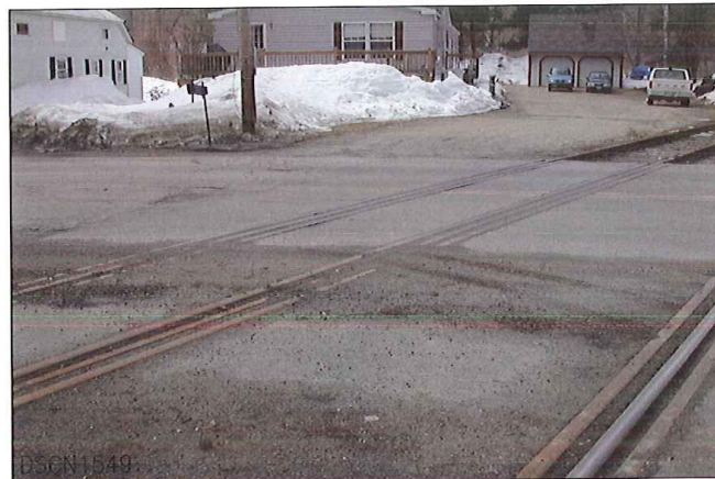
LOOKING FROM EAST TO SIDE TRACK
