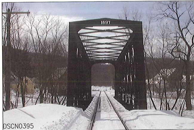
BACK RIVER BRIDGE
