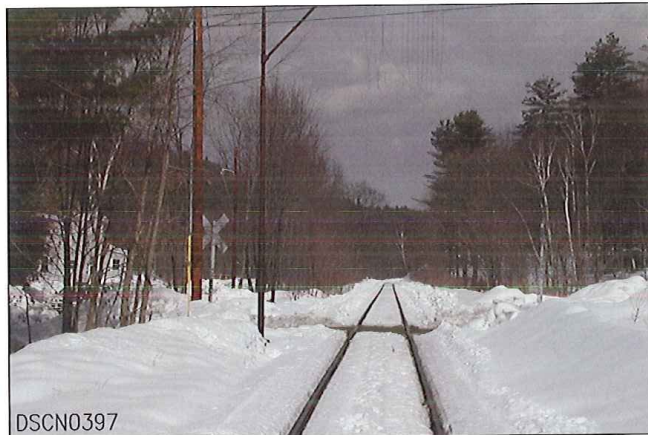
LOOKING FROM WEST TO EAST
