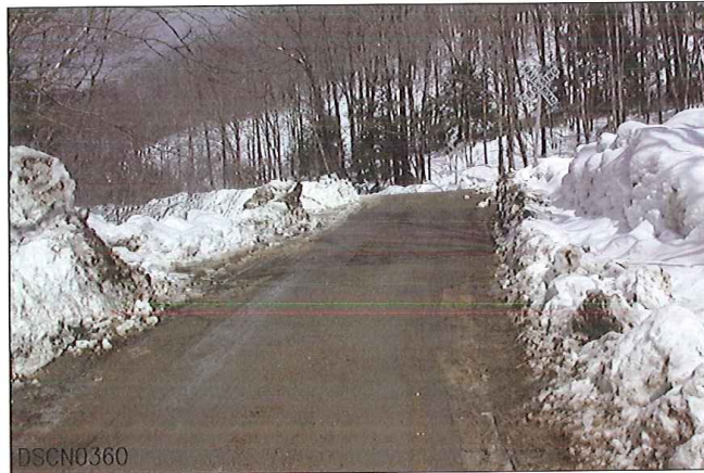
LOOKING FROM SOUTH TO NORTH
