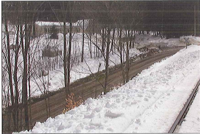
LOOKING FROM WEST TO NORTH
