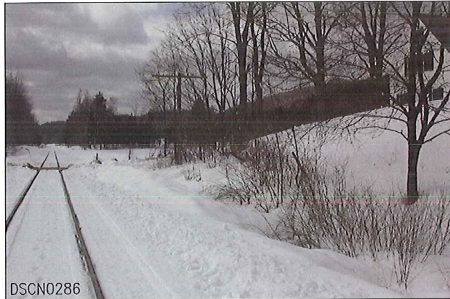
LOOKING FROM WEST TO SOUTH
