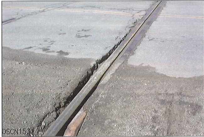
LOOKING FROM EAST TO WEST, SOUTH RAIL
