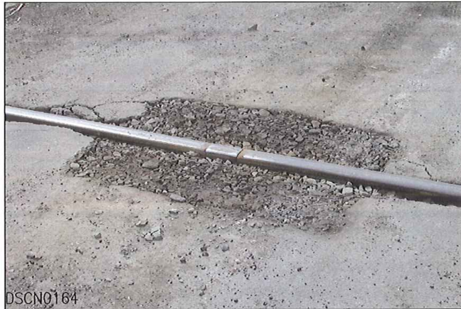
SOUTH RAIL – DUTCHMAN INSTALLED
