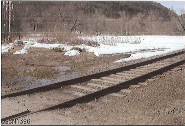
LOOKING TO NORTHWEST QUADRANT
