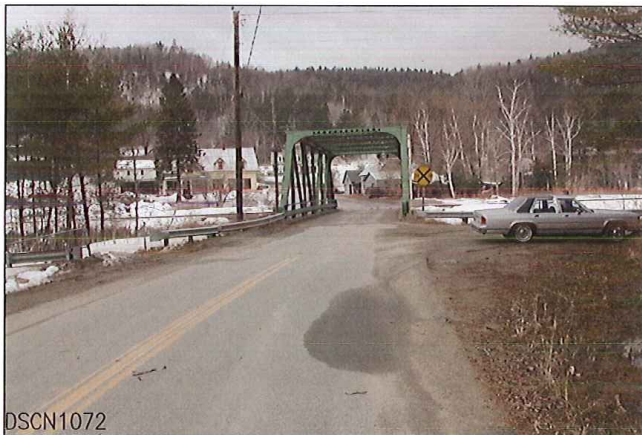
LOOKING FROM WEST TO EAST
