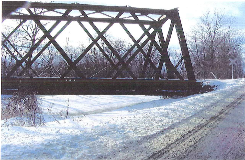
Picture No. 52 Looking Northwest, Bridge 229 Crossing, Leicester, VT
