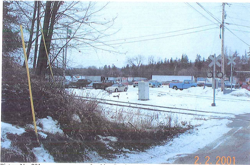
Picture No. 291 Looking Southwest, Depot Lane Crossing, Rutland Town, VT
