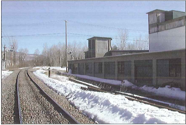
LOOKING FROM WEST TO SOUTH
