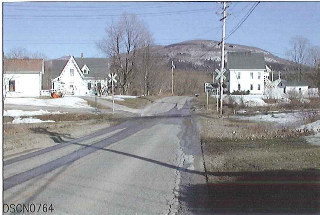
LOOKING FROM SOUTH TO NORTH
