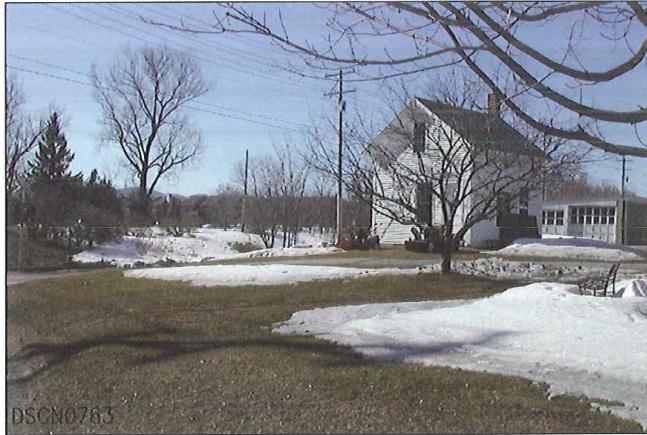
LOOKING FROM NORTH TO WEST
