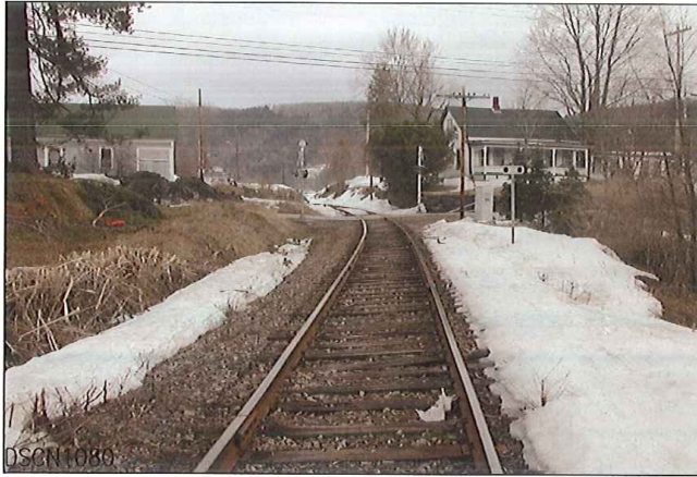
LOOKING FROM SOUTH TO NORTH
