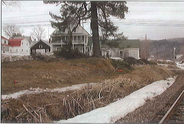
LOOKING FROM SOUTH TO WEST
