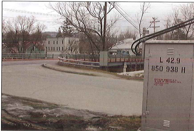
LOOKING FROM SOUTH TO EAST
