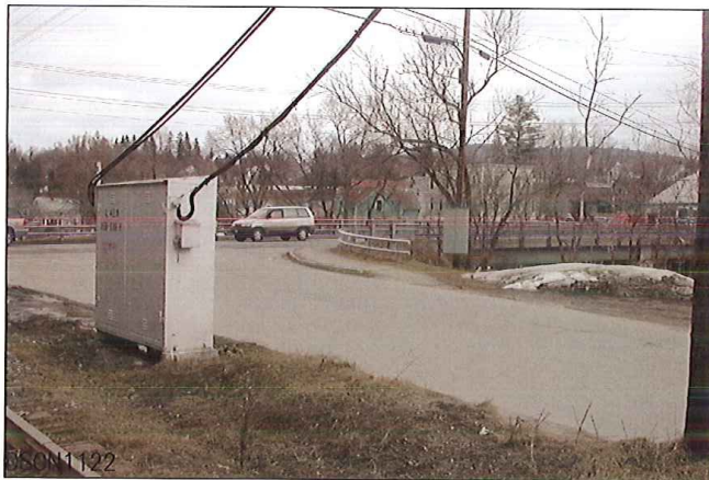
LOOKING FROM SOUTH TO EAST
