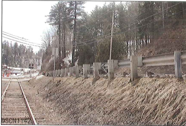
LOOKING FROM NORTH TO WEST
