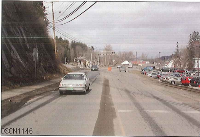
LOOKING FROM WEST TO EAST
