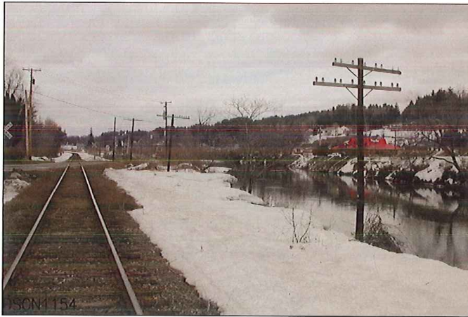
LOOKING FROM SOUTH TO EAST
