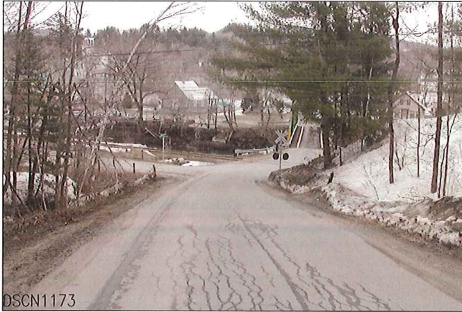
LOOKING FROM WEST TO EAST
