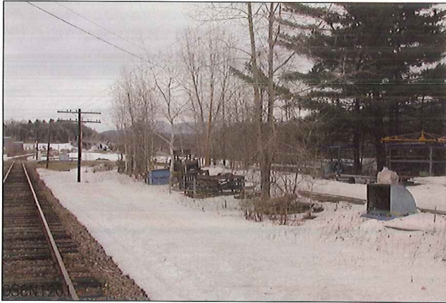
LOOKING FROM SOUTH TO EAST
