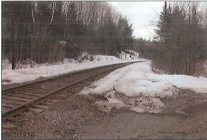
LOOKING FROM WEST TO SOUTH
