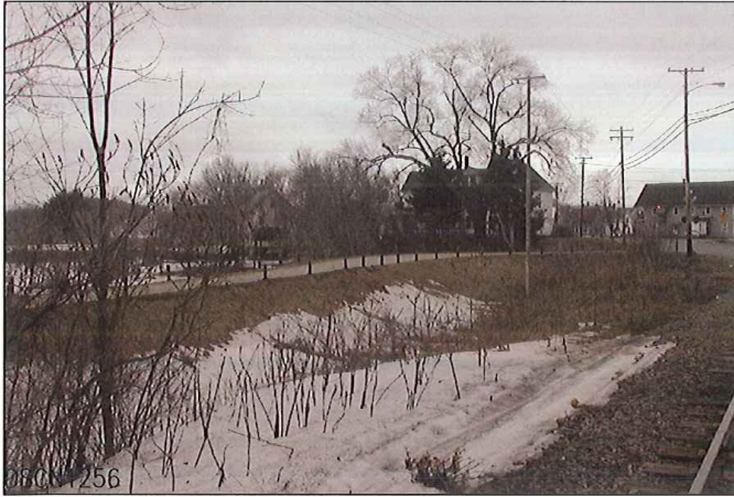
LOOKING FROM SOUTH TO WEST
