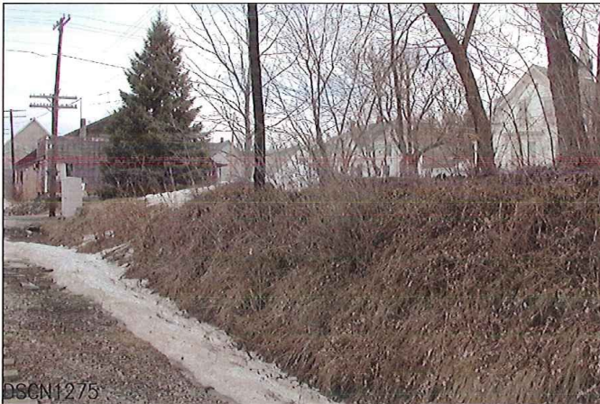
LOOKING FROM SOUTH TO EAST
