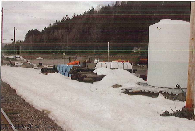
LOOKING FROM NORTH TO WEST
