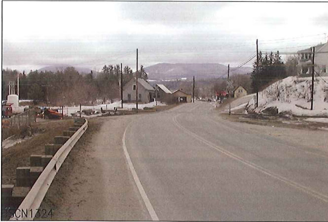
LOOKING FROM WEST TO EAST
