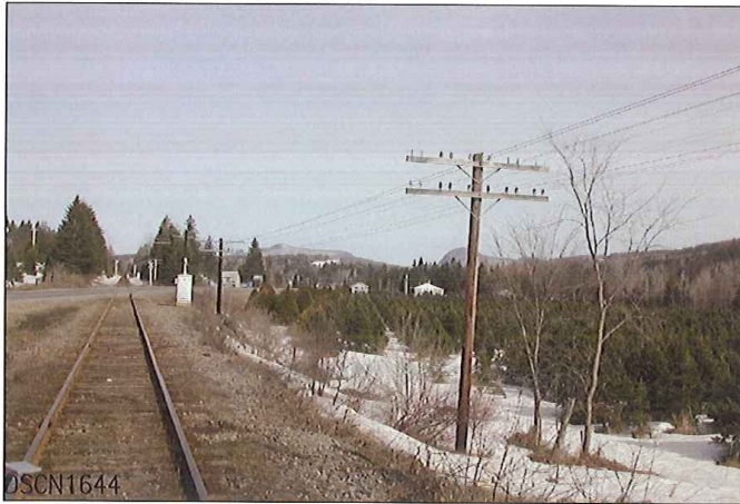
LOOKING FROM SOUTH TO EAST
