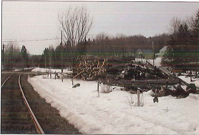
LOOKING FROM NORTH TO WEST
