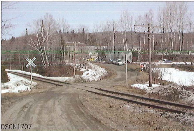
LOOKING FROM WEST TO EAST
