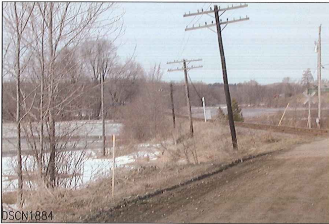
LOOKING FROM WEST TO NORTH
