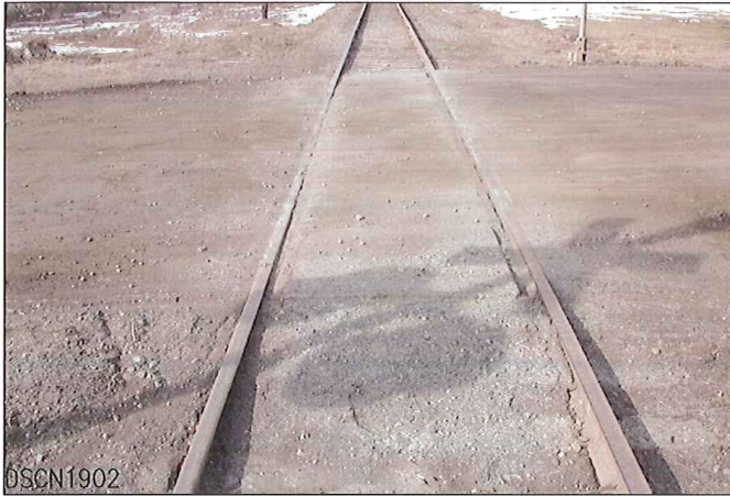
LOOKING FROM SOUTH TO NORTH
