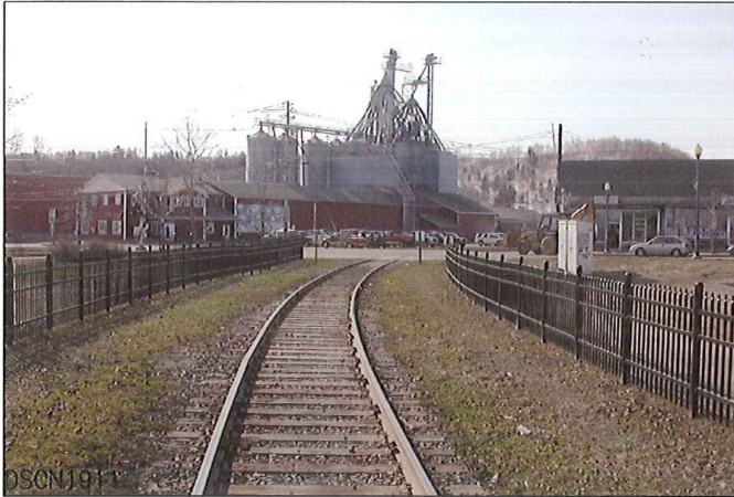
LOOKING FROM NORTH TO SOUTH – MAINLINE
