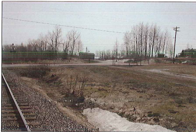
LOOKING FROM NORTH TO WEST
