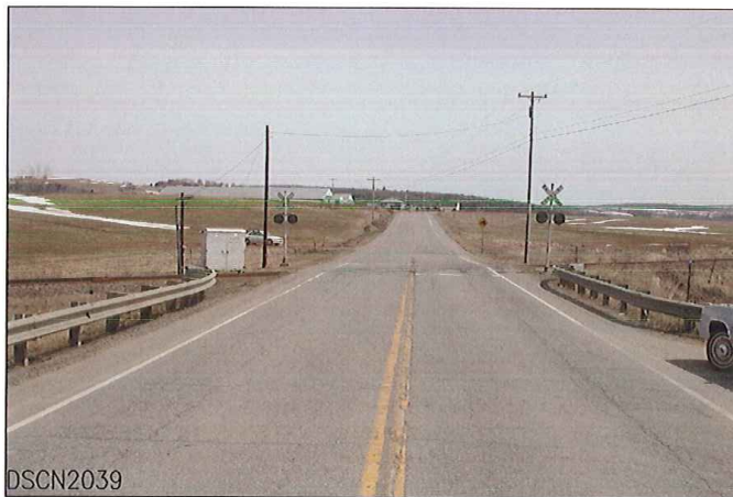
LOOKING FROM WEST TO EAST
