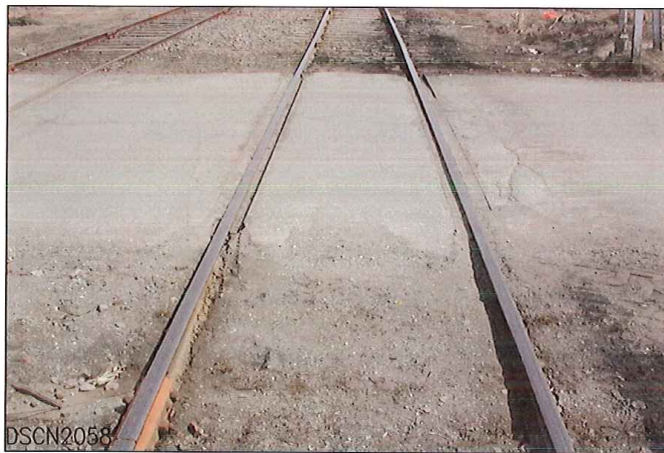
LOOKING FROM NORTH TO SOUTH – MAINLINE
