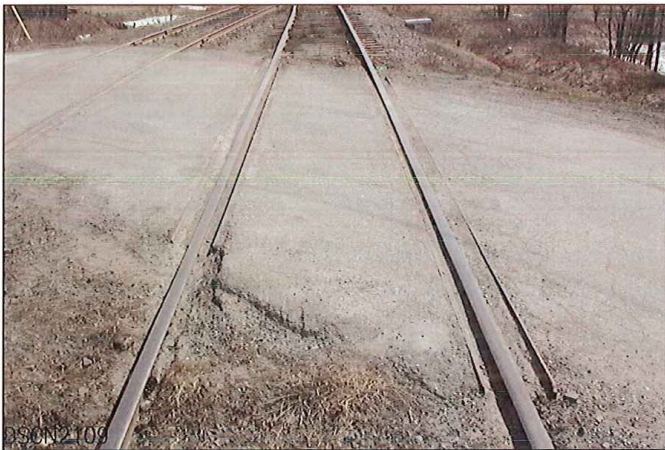
LOOKING FROM NORTH TO SOUTH MAINLINE
