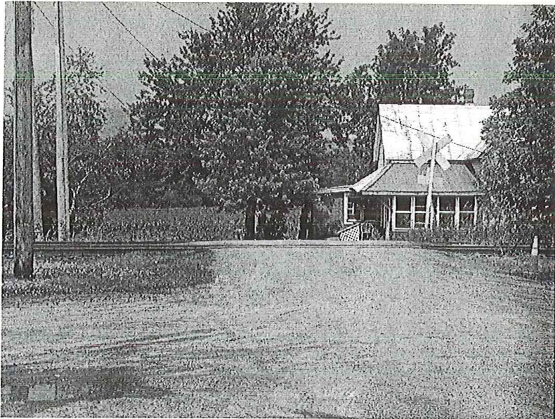
RICHFORD 847-868S VIEW FROM EAST TO WEST JULY 21, 2004
