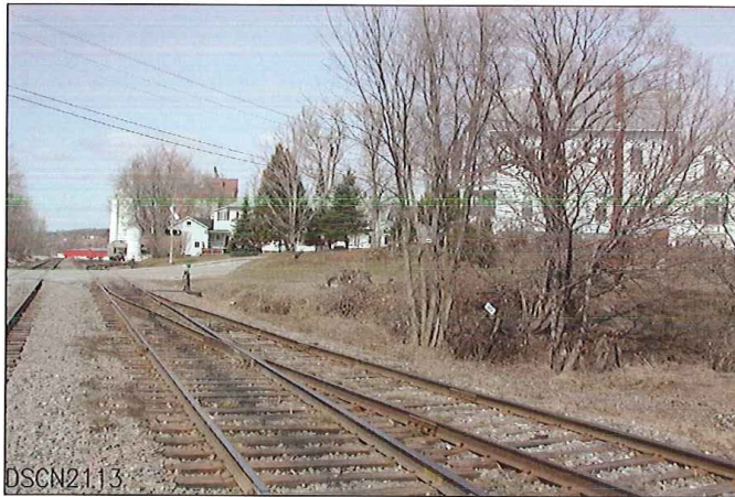
LOOKING FROM SOUTH TO EAST
