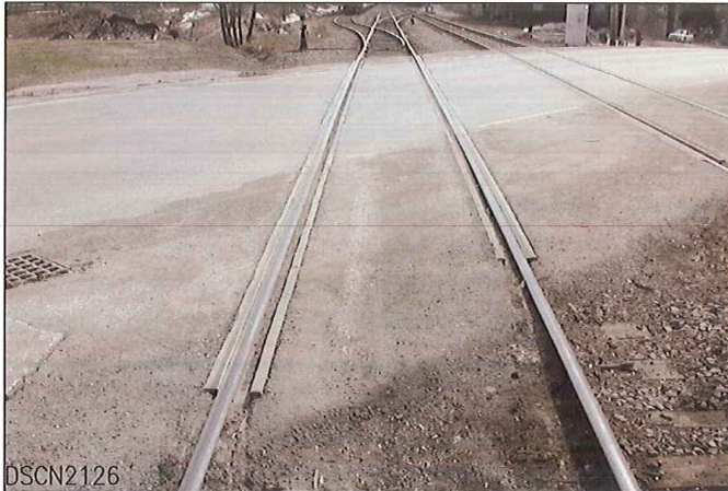
LOOKING FROM NORTH TO SOUTH SIDETRACK
