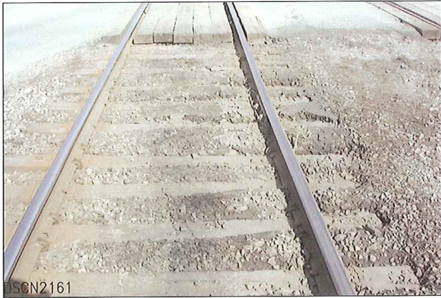
LOOKING FROM SOUTH TO NORTH – MAINLINE TRACK
