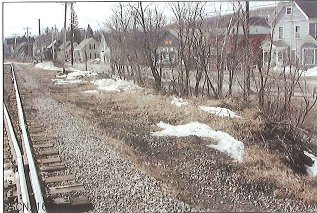
LOOKING FROM NORTH TO WEST
