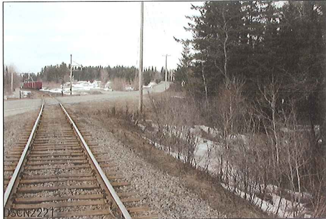
LOOKING FROM SOUTH TO EAST
