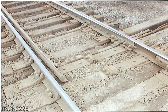
SWITCH NORTH OF CROSSING
