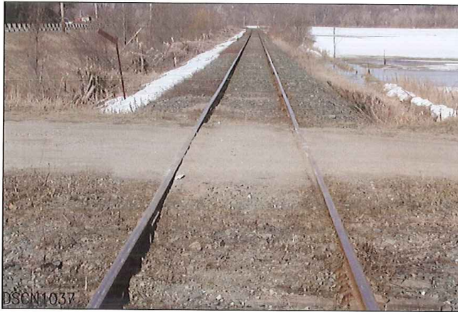
LOOKING FROM SOUTH TO NORTH
