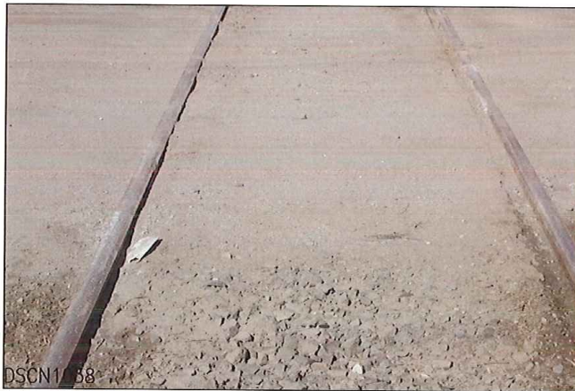
LOOKING FROM SOUTH TO NORTH
