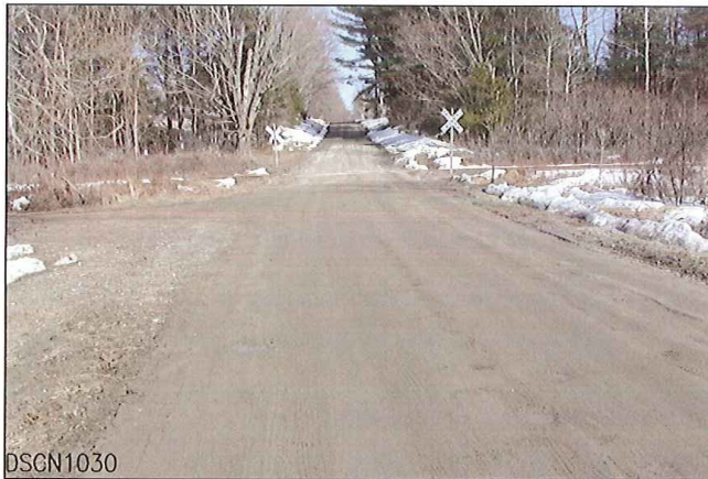
LOOKING FROM WEST TO EAST
