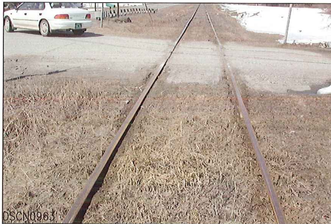
LOOKING FROM SOUTH TO NORTH
