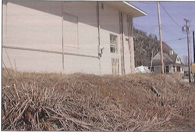
LOOKING FROM SOUTH TO WEST
