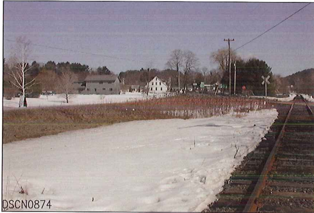
LOOKING FROM SOUTH TO WEST
