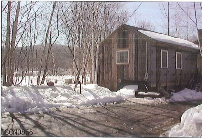
LOOKING FROM WEST TO SOUTH
